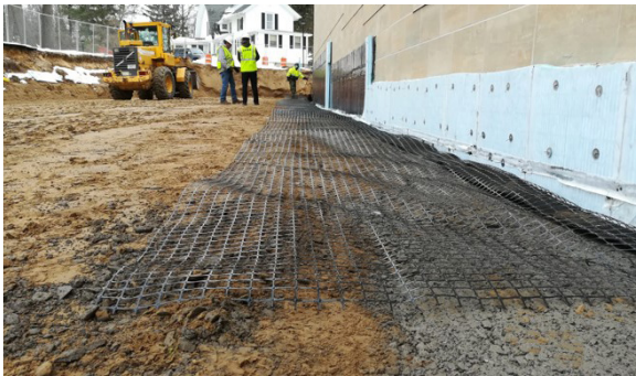
Approaching finished grade
