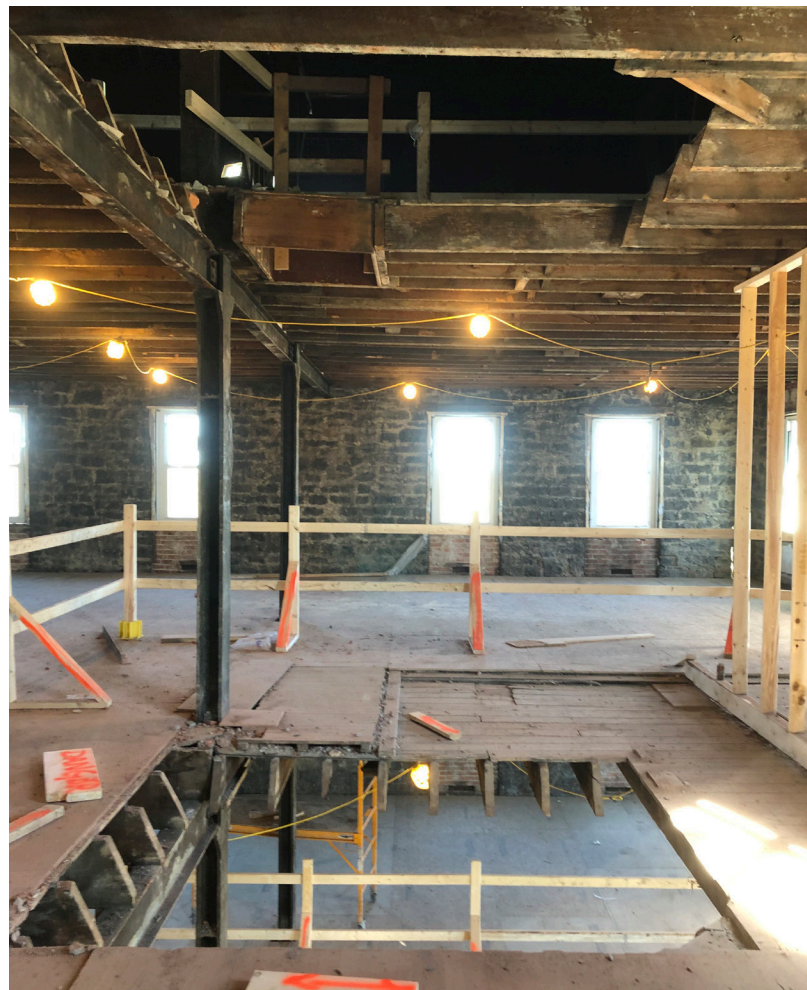
Demolished elevator shaft requiring infill framing
