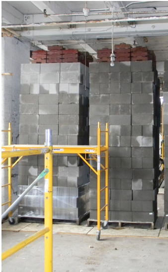
Load test to verify capacity of the existing floor framing
