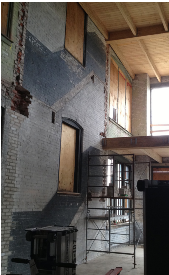
Removal of an existing stair shaft requiring modification of the floor framing (in-progress)
