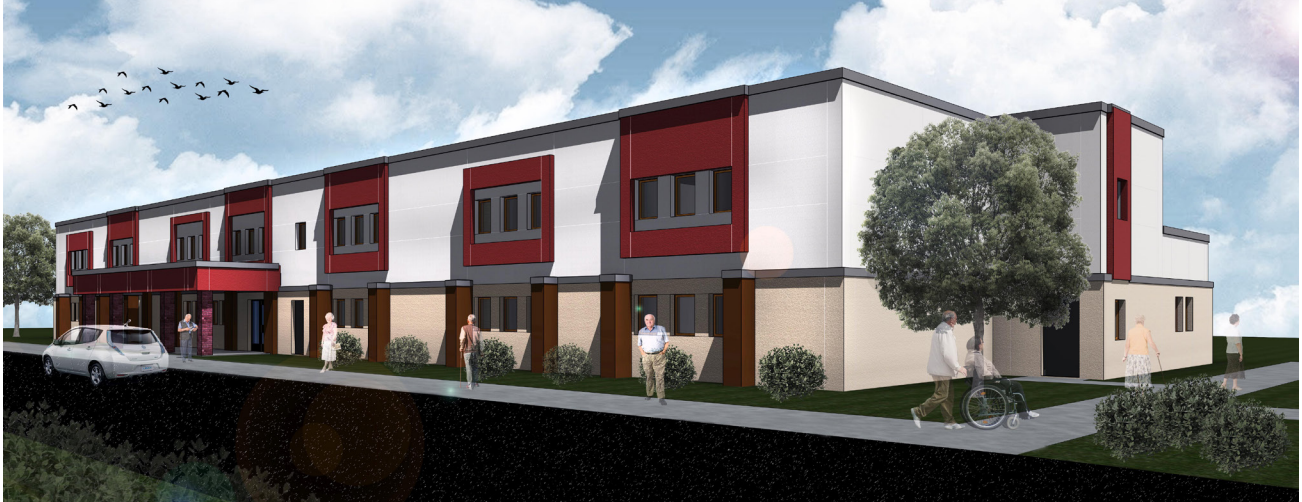
RetrofitNY is leading the effort to create design solutions to renovate and modernize their test pilot projects, as shown above.
