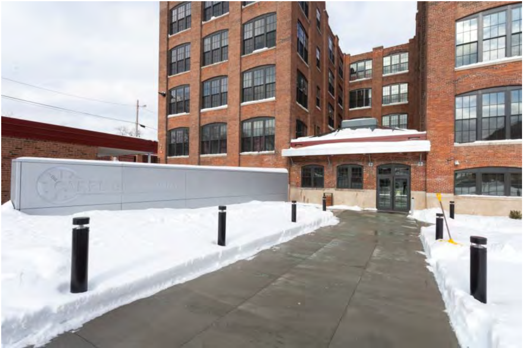
Carriage Factory Apartments new entrance signage, focal wall and entrance canopy to the building
