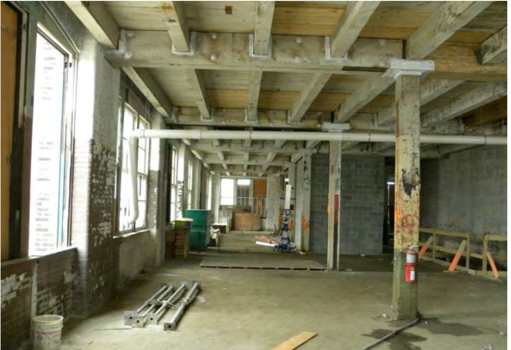
Existing conditions of the interior before restoration
