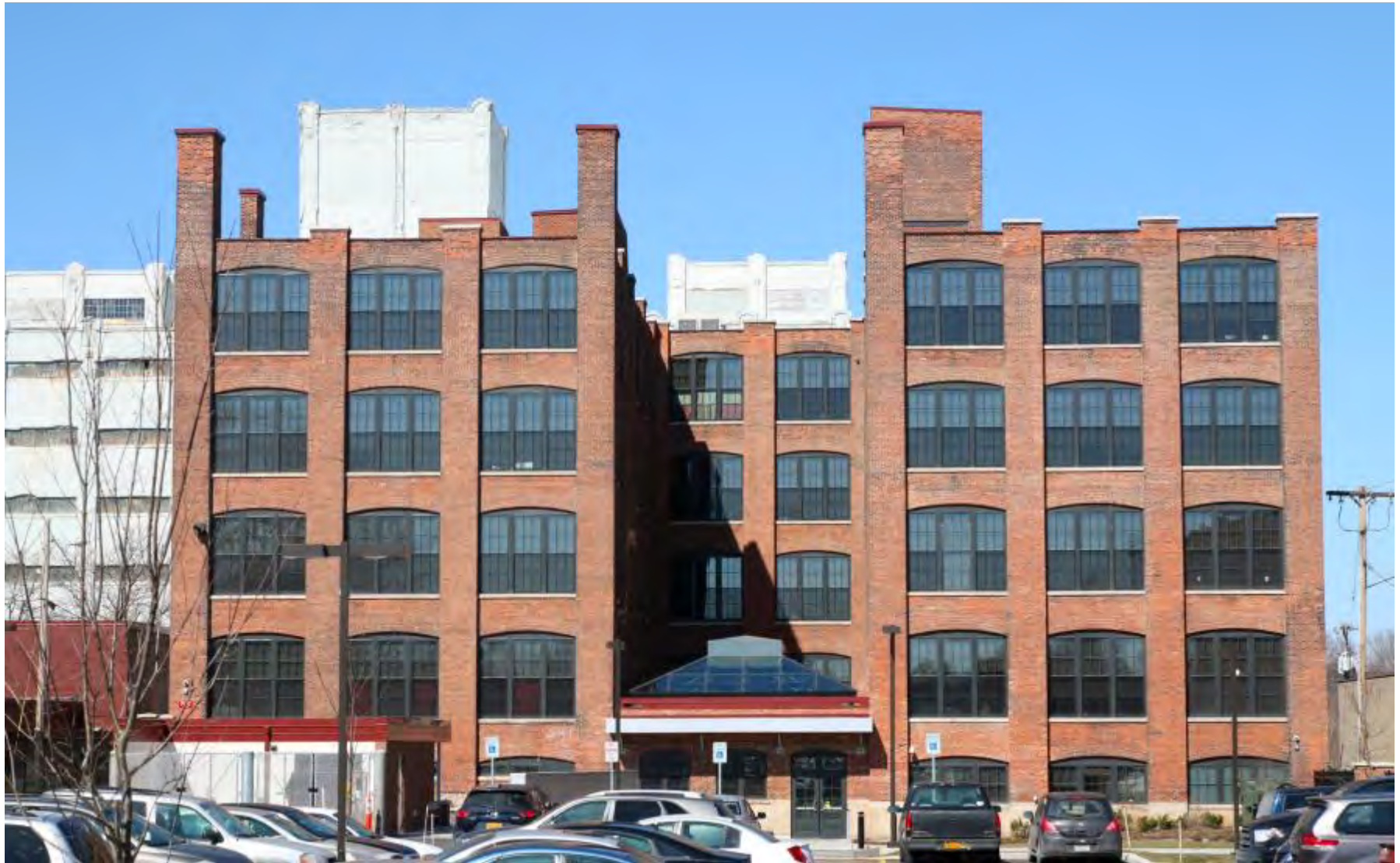
Restored entrance to the Carriage Factory Apartments including brick re-pointing and structural repairs to the exterior masonry
