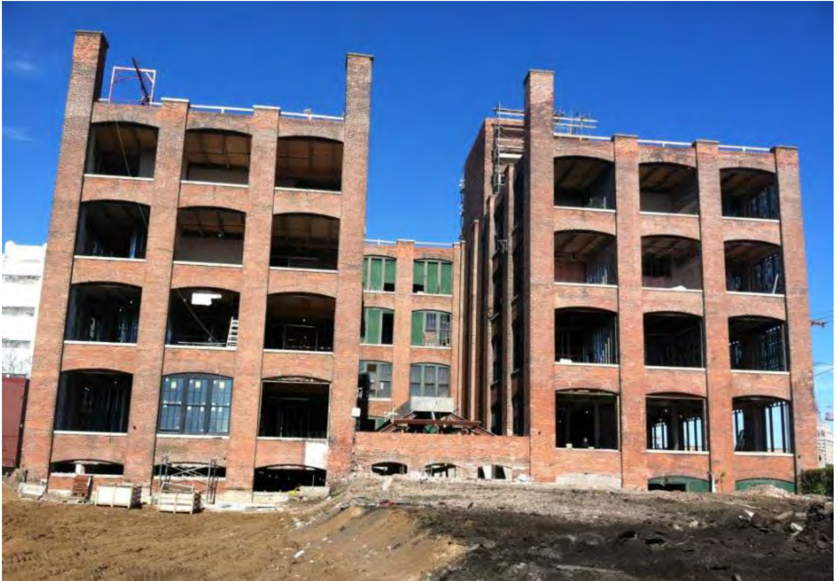
The large exterior single pane hung windows of the building were in great disrepair and required complete replacement
