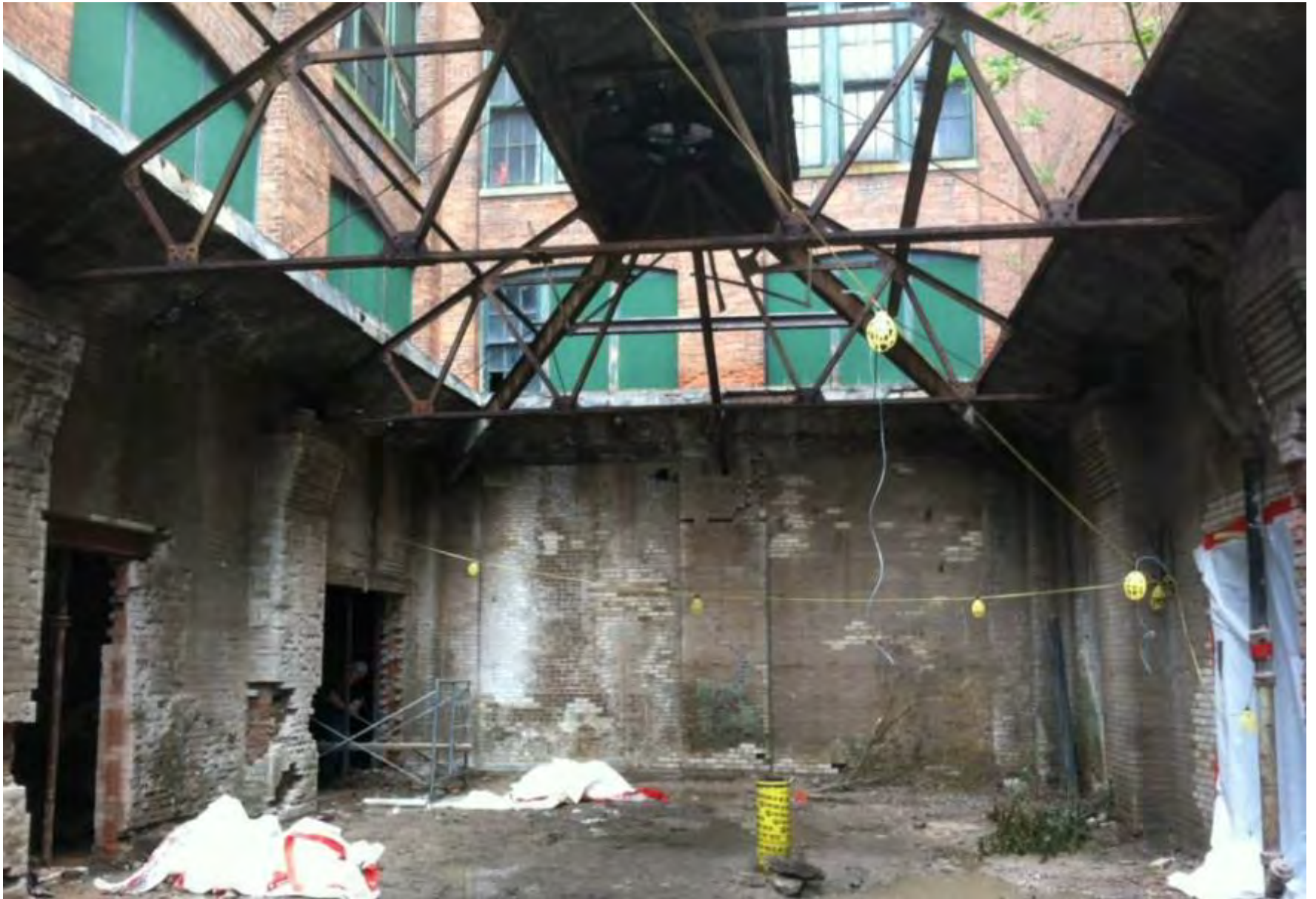
Existing glass skylight was boarded up and the exposed steel trusses rusted in many locations
